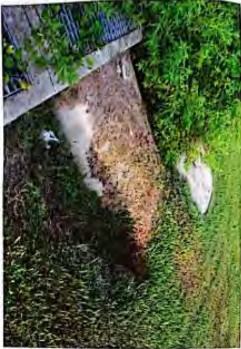
Erosion between pipes at Control Structure south side of 58th St E
