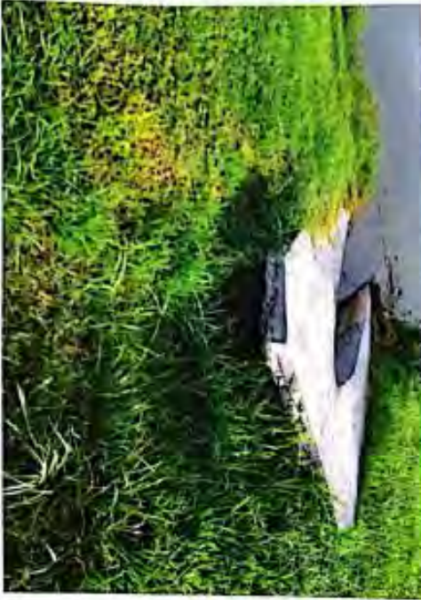
Erosion between pipes at Control Structure south side of 58th St E
