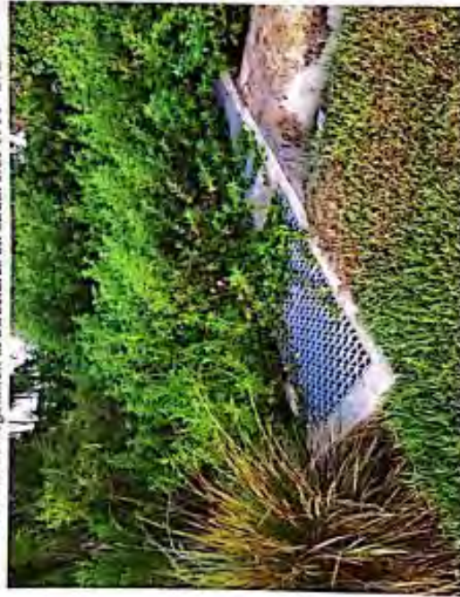
Excessive vegetation at Structures on south side of 58 th St E
