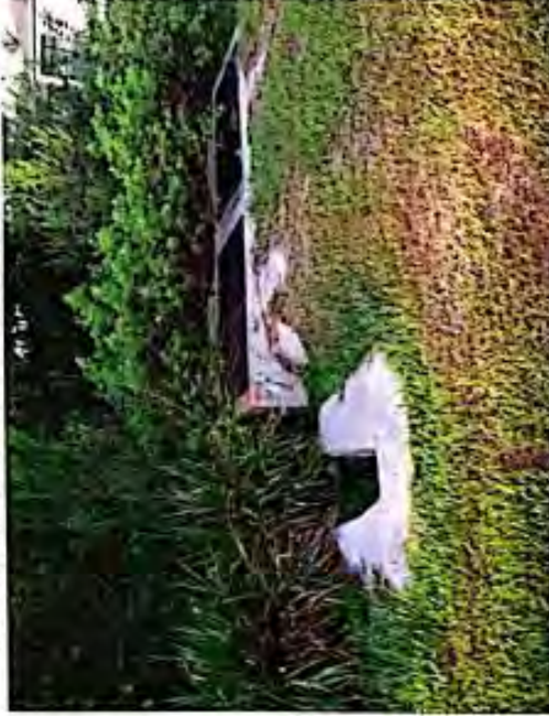
Erosion behind center of MES on north side of 110 th Ave East
